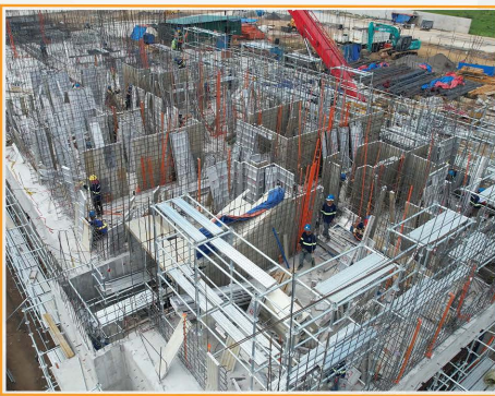
Exterior & Interior Walls
